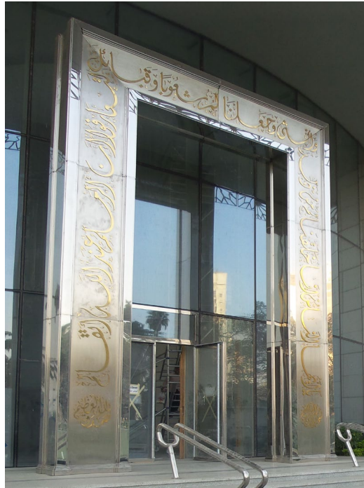
Fence, Claddings & Staircases – Embassy of KSA
