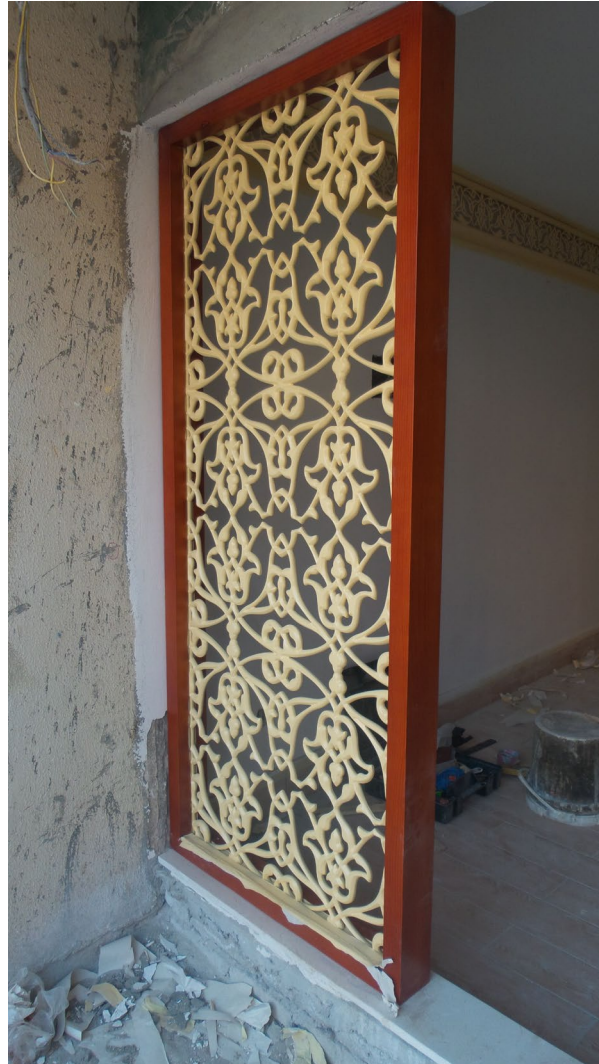
Wooden Partitions & Ceiling Claddings – Marriot Zamalek
